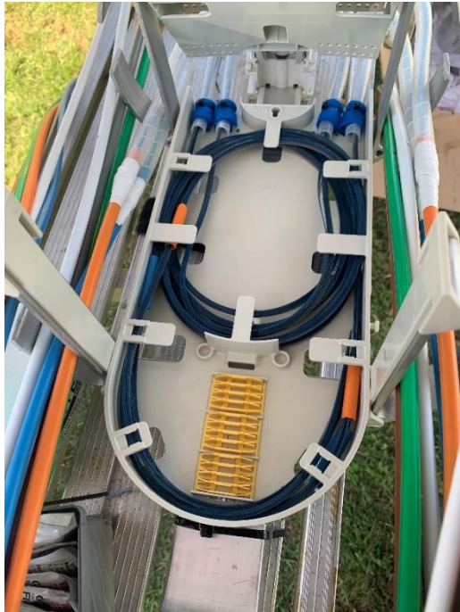
Figure 13 - First tray with 2 flat ribbon tubes looped and stored for further cleaning and splicing
