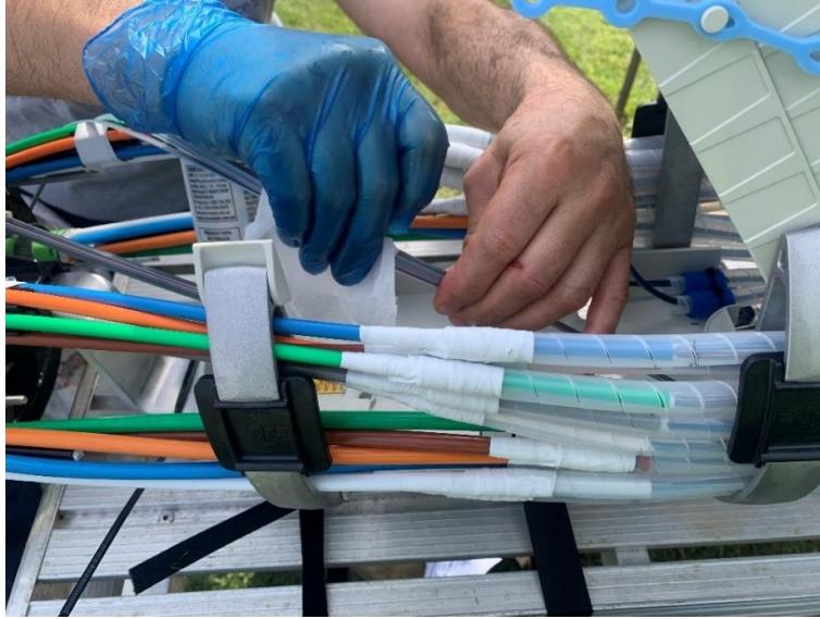
Figure 20 - Flat ribbons having the gel cleaned by wiping and applying isopropanol
