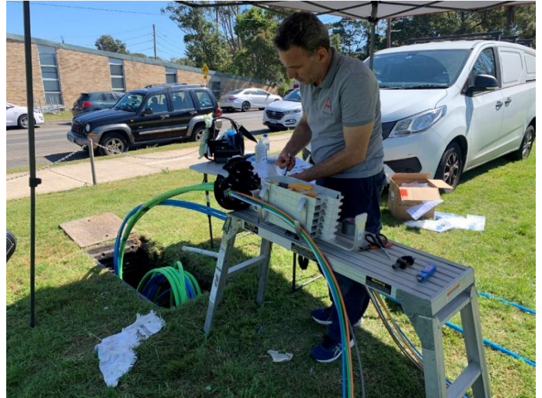
Figure 11 - Fitting the first cable into the COYOTE® HD Dome Closure
