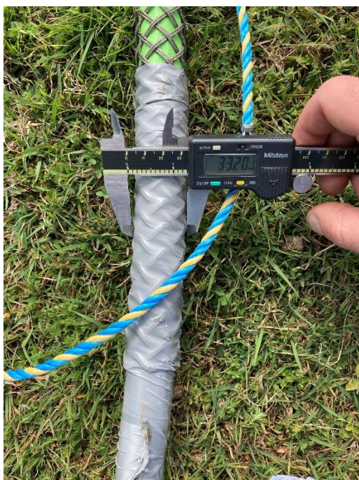
Figure 4 - Flat ribbon cable diameter measured with the hauling sock fitted
