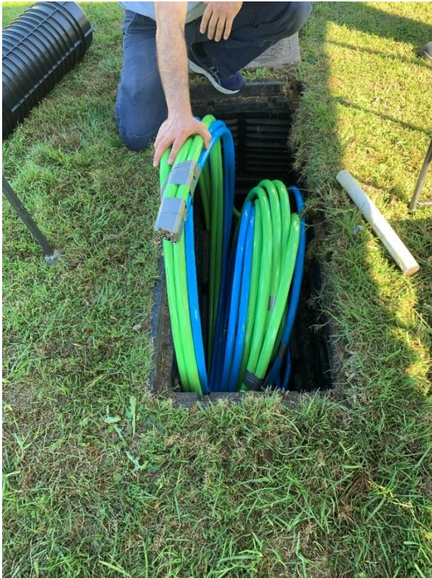
Figure 12 - Ribbon cables taped together, coiled and cut to the correct length to enter the closure
