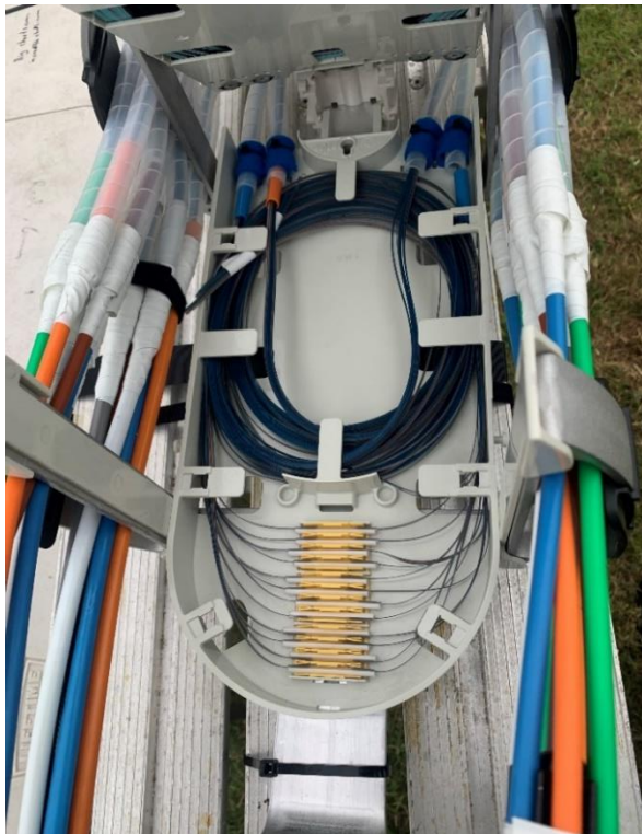
Figure 22 - Photo of the first flat ribbon tube fully spliced on the closure tray
