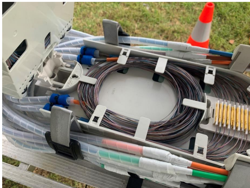
Figure 23 - Photo of the first 2 FlexRibbon™ tubes on the closure tray
