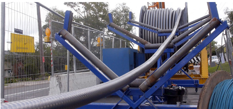
Clockwise from top left: Prysmian 132 kV XLPE cable being prepared for installation; Prysmian 132 kV outdoor terminations to be connected to Ausgrid network; cable installation into existing Ausgrid substation; progressive installation of Prysmian 132 kV cable.
